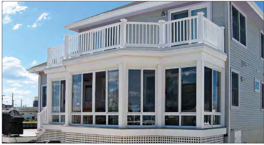
This Elite sunroom located on the Jersey Shore withstood the 140 mph winds of Hurricane Sandy without damage.
