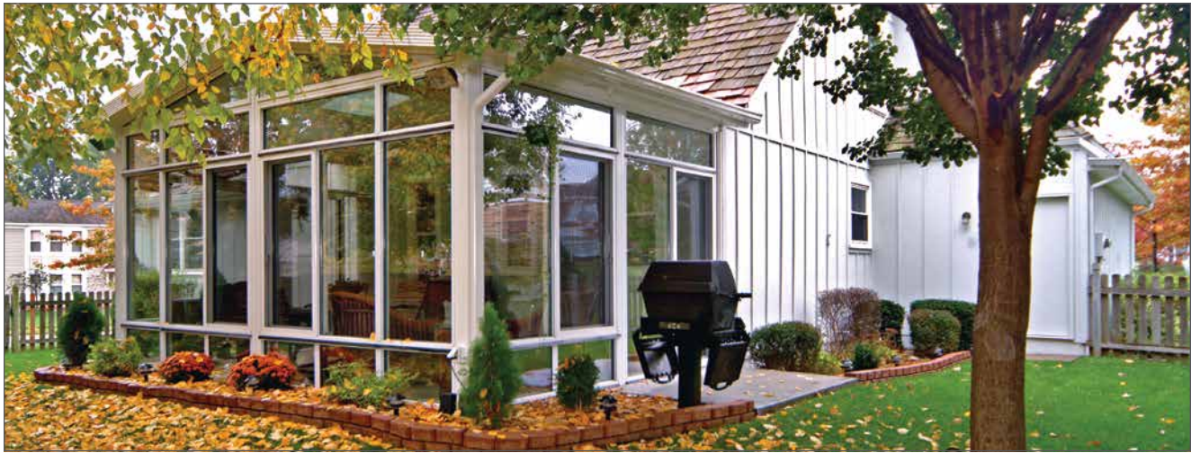
The changing seasons are enjoyed in this gabled-roof sunroom with glass wing, glass knee wall and a transom for expansive views and maximum natural light.
