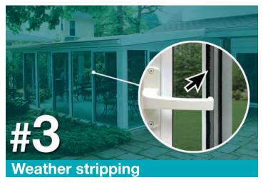
Weather stripping is the barrier designed to keep out the elements.
