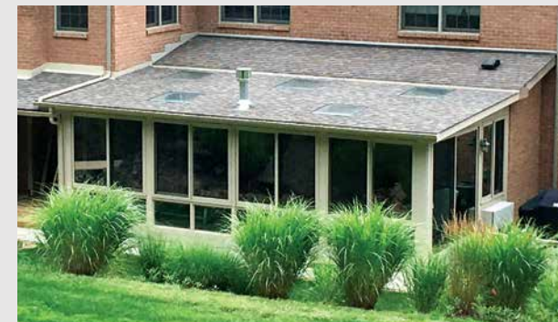
Glass roof panels flush with the roof prevent ice and snow build-up.
