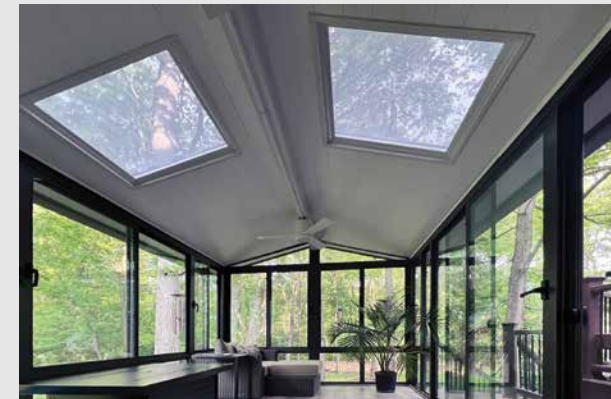
Removable screens on 3'x3' roof panels control incoming light.
